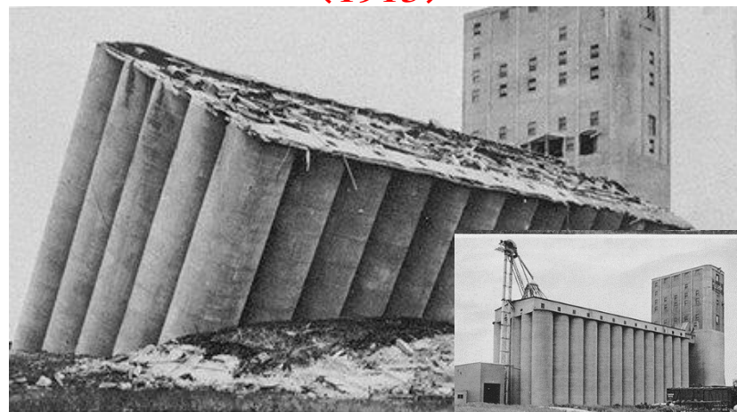
Transcona Grain Elevator (1913)
